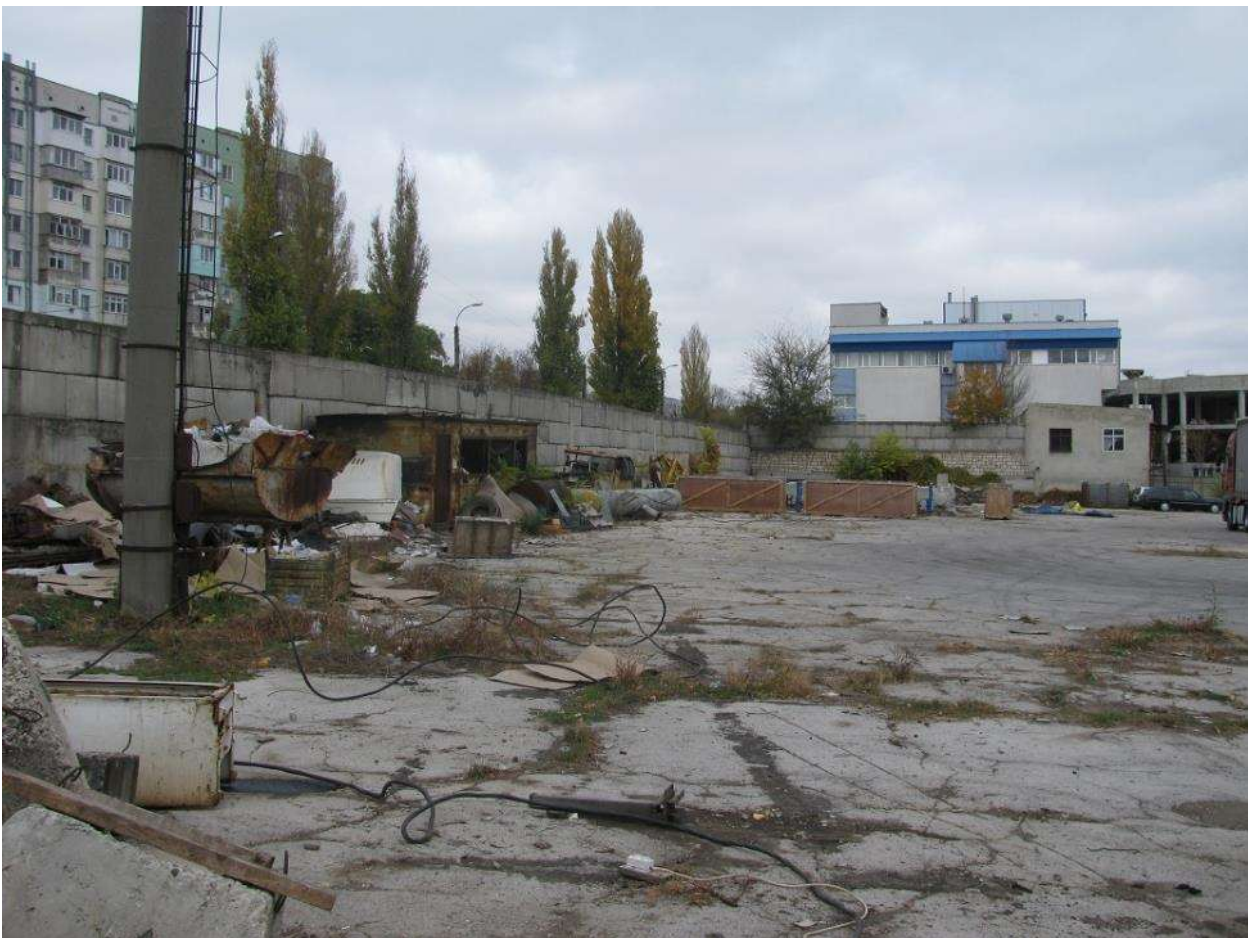
Photo 1: Selected site for new ME building (Nov 2018).
