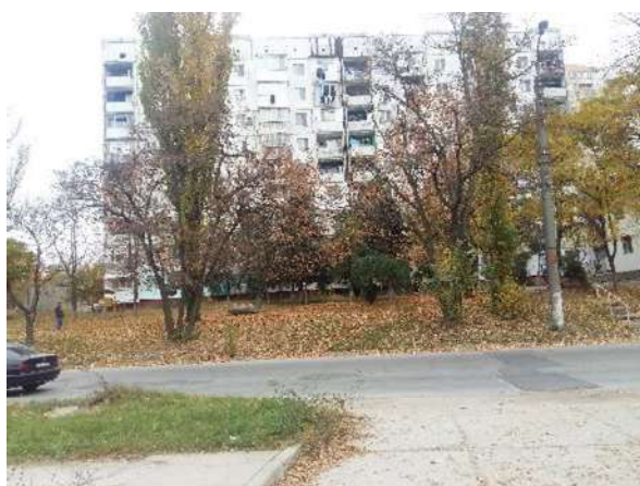
Multistore building – western part, 50 m far from project location
